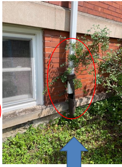
Bad Location to drain water from the roof top
