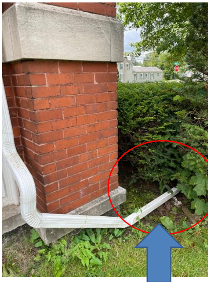
Bad Location to drain water from the roof top
